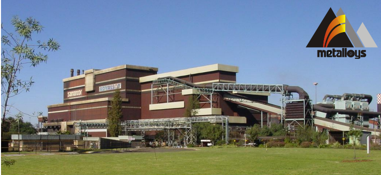
Samancor Metalloys, West Plant - Meyerton, Gauteng, South Africa
