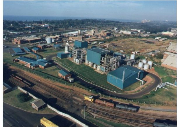
SABioproducts Lysine Manufacturing Plant Umbogintwini, Kwa-Zulu Natal coast, South Africa
